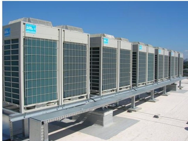
Figure 17: Central system VRF pilot building #2
