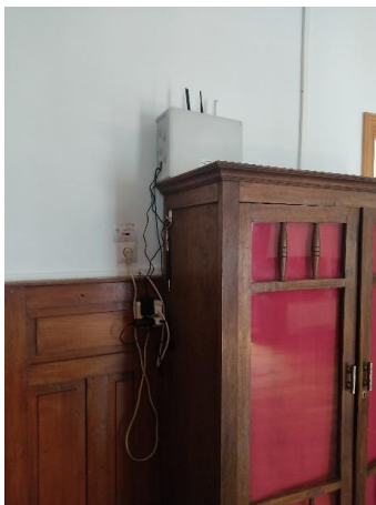
Figure 89. Concentrator for data reception in DS7. May 22th 2024.
