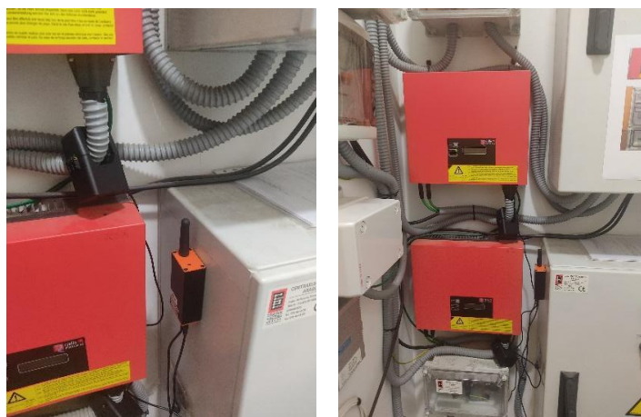
Figure 96. Measurement of the output of the PV system at the inverter in DS7. June 6th 2024.
