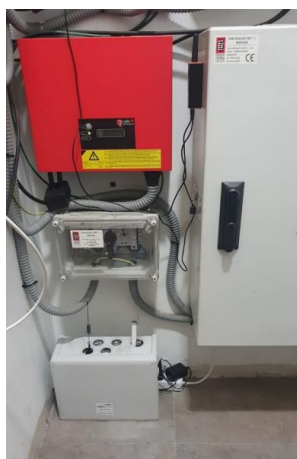
Figure 98. Installation of a new concentrator for data reception in DS7. August 2nd 2024.
