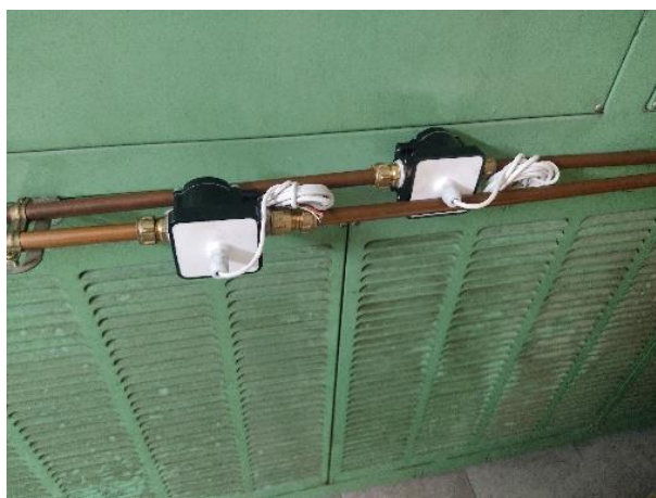
Figure 90. Fuel oil meters in boiler and HVAC system in DS9. June 4th 2024.
